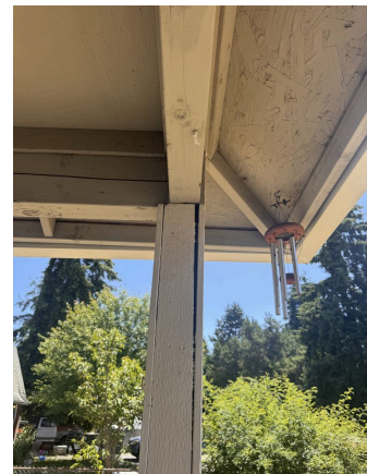
Trim covering framing is loose.
