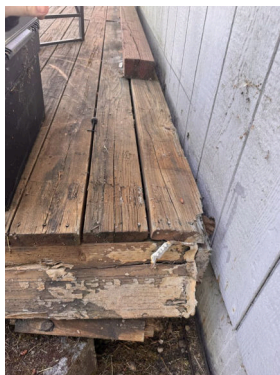
Improper attachment
