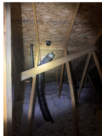
Laundry room duct
